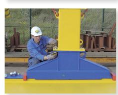
Depending on the trench width, flange the strut extensions onto the rolling struts.
