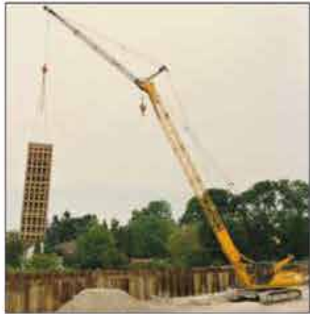
1976-1995: S 1225 crawler crane with fly boom to lift casing boards
